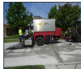
2015 Photos of the milled roadways with detail 7 joint repairs and scratch course The FiberMat® consisted of
