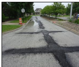
2015 Photos of the milled roadways with detail 7 joint repairs and scratch course The FiberMat® consisted of
