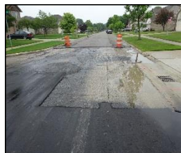
2015 Photos of the milled roadways with detail 7 joint repairs and scratch course The FiberMat® consisted of
