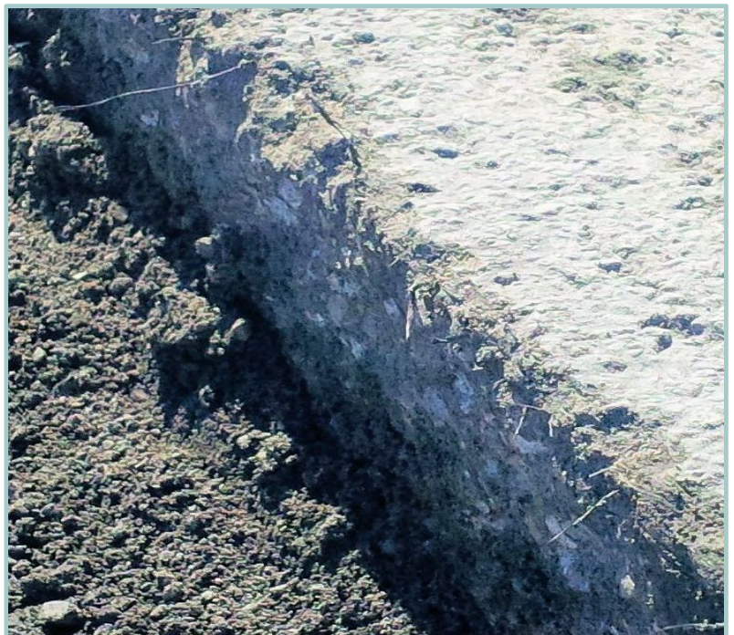
FiberMat® still in place after 7 years
