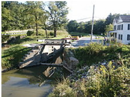
Restored Ohio & Erie Canal Lock
